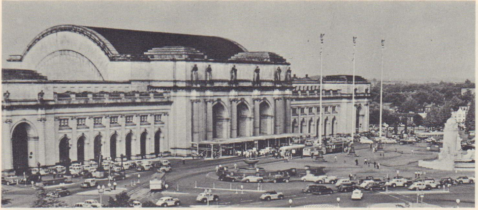
UNION STATION: Union Station, Washington, D. C., where all lines into the nation's capital meet in a single terminal.
